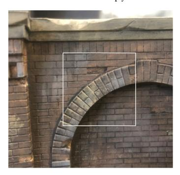
The sample approx. 80\*80 cm, must include a missing brick, the standard horizontal brickwork and a section of the protruding arch.
